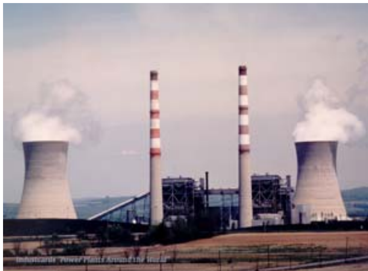
Montour Power Plant
