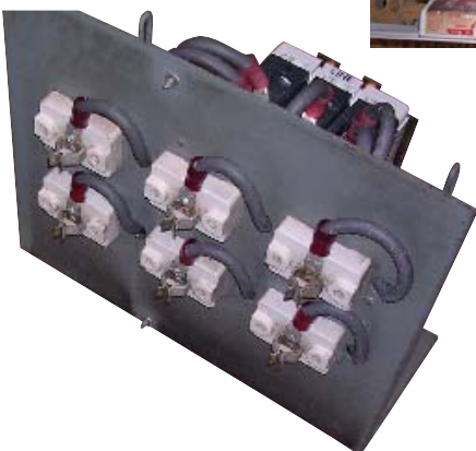
Custom design to accommodate dual stabs to increase amperage on a very old GE MCC.
