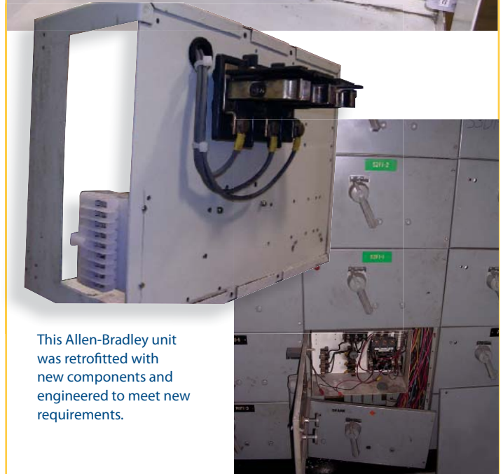
Custom design to accommodate dual stabs to increase amperage on a very old GE MCC.
