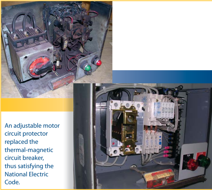
Complete retrofitted units are easily installed in the old MCC structures.
