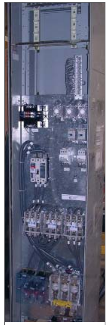
Custom size 5 vacuum multi-speed starter
