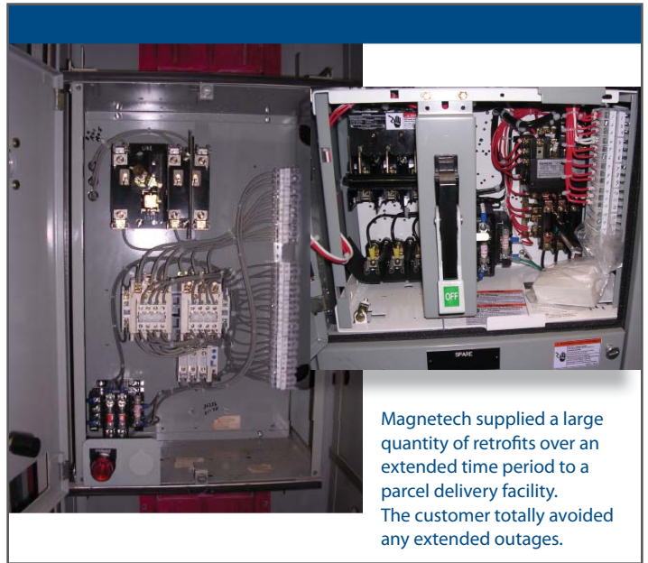
Two speed, two winding, vacuum starter with all the bells and whistles.
