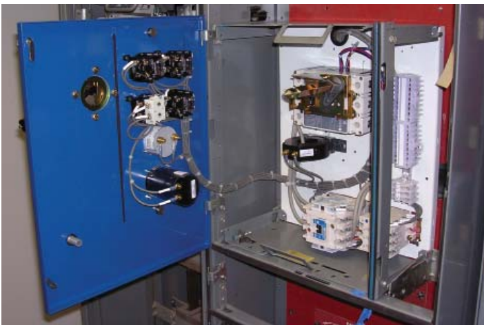
Several C-H F-10 units with a complicated device panel were retrofitted for a large auto manufacturer.
